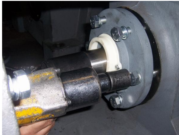
Figure 48 Worm Shaft Bearing replacement
