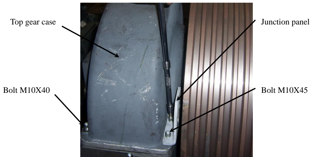
Figure 29 Reinstall Junction panels
