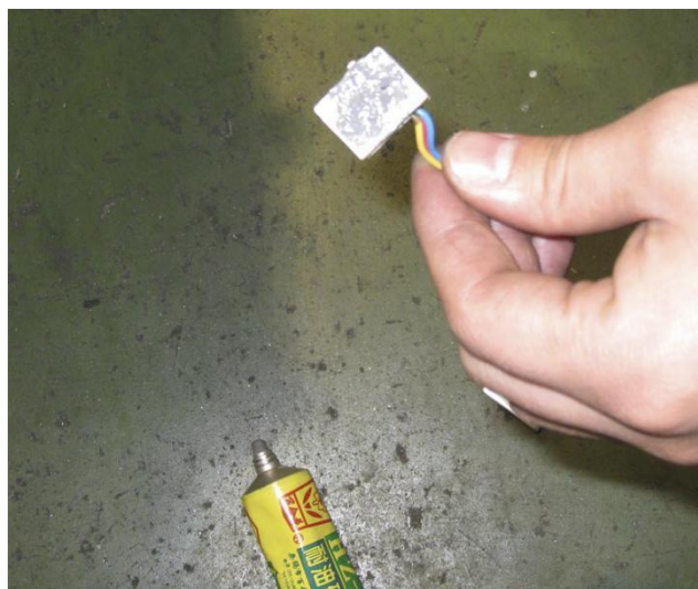
Figure 27: Applying sealant to brake switch
